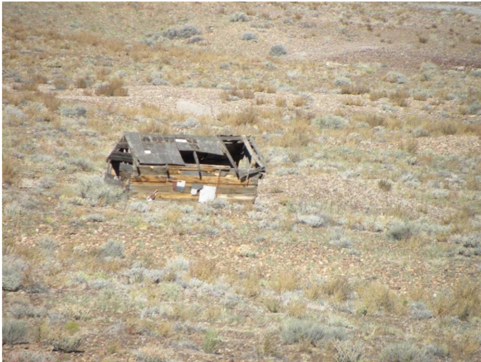
Photo 3. Charles Huskon No. 14 mine site, nearby collapsed wood structure
