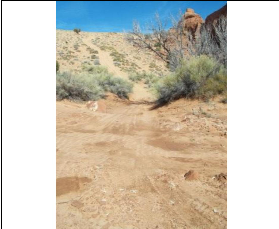
Photo 1 Impassable road in direction of the site
