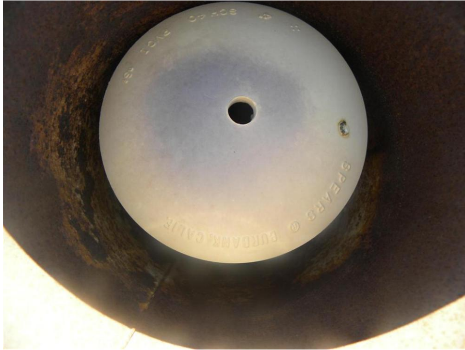
Photo 9. New Liba Group, Site #522, PVC tube inside metal casing
