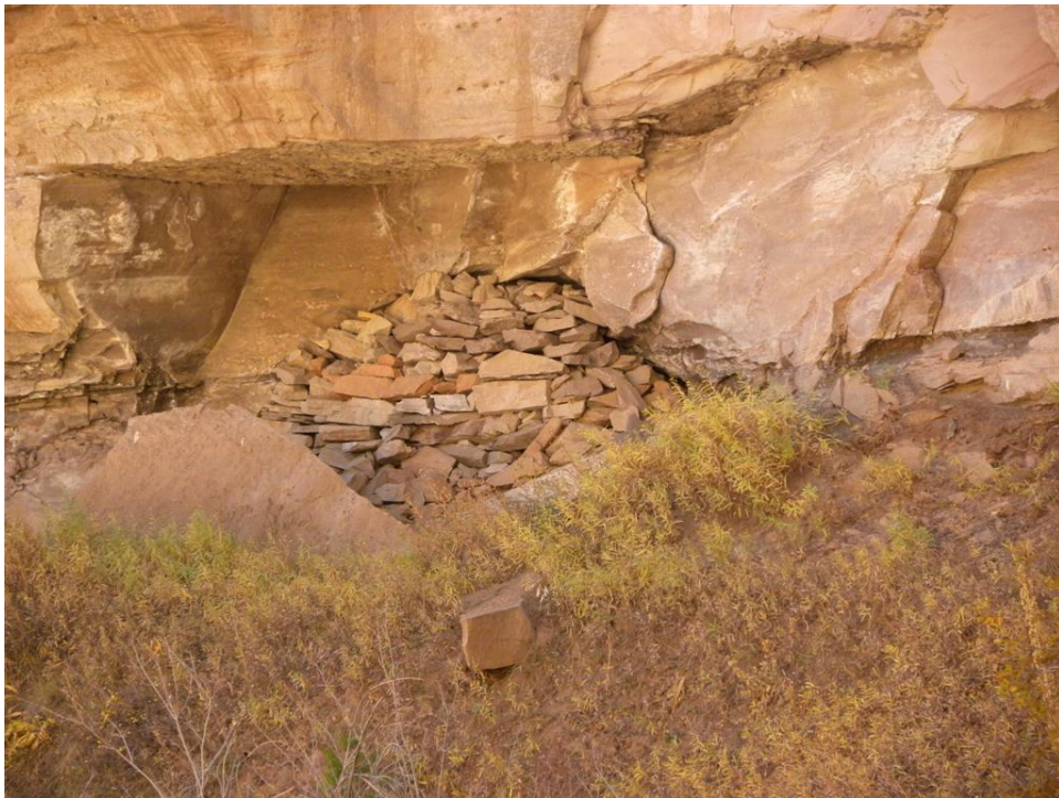
Photo 12. Mine site #612 sealed adit
