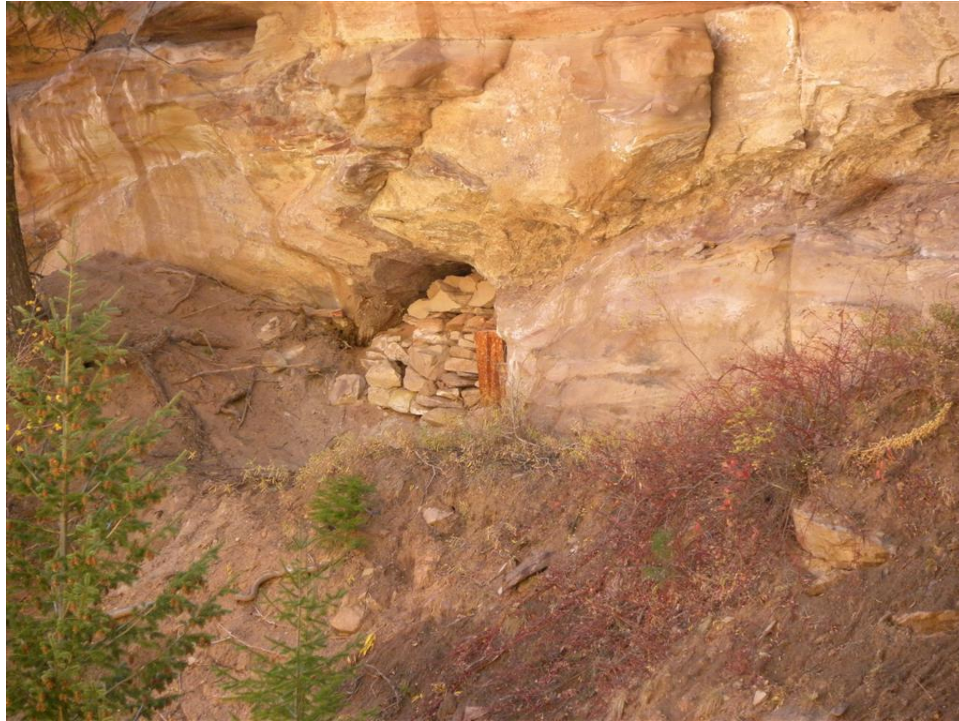
Photo 13. Mine site #612 sealed adit
