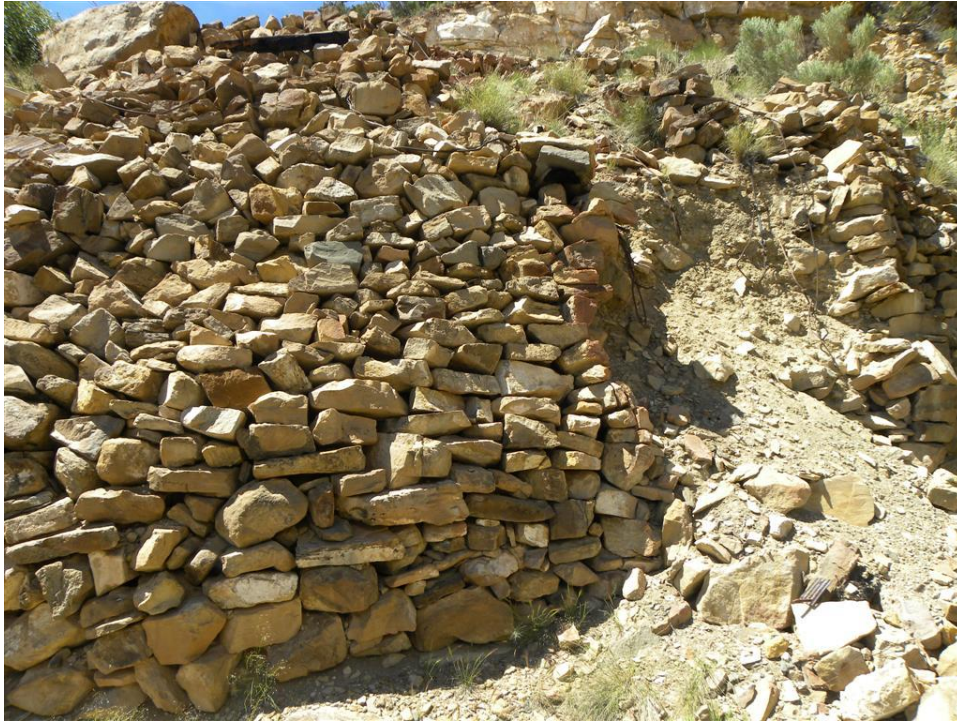
Photo 3. Tony Tuc site, sealed adit
