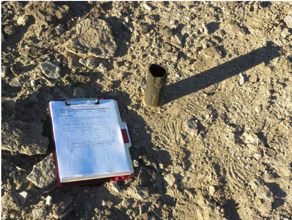
Photo 4. Charles Huskon No. 26 mine site, protruding casing
