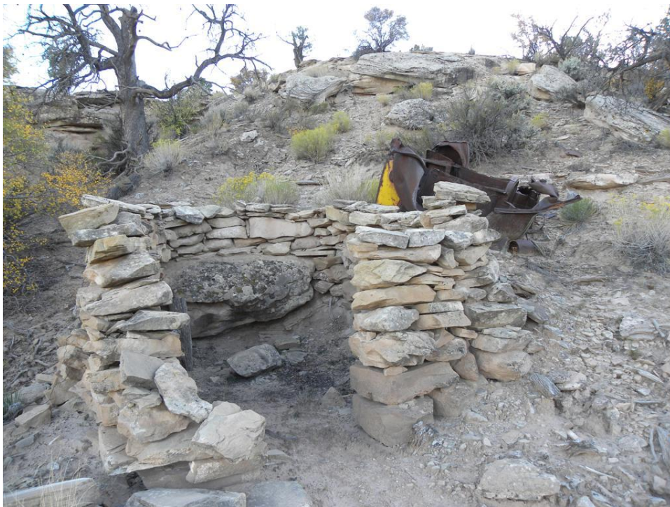
Photo 6. Stacked rock and metal debris
