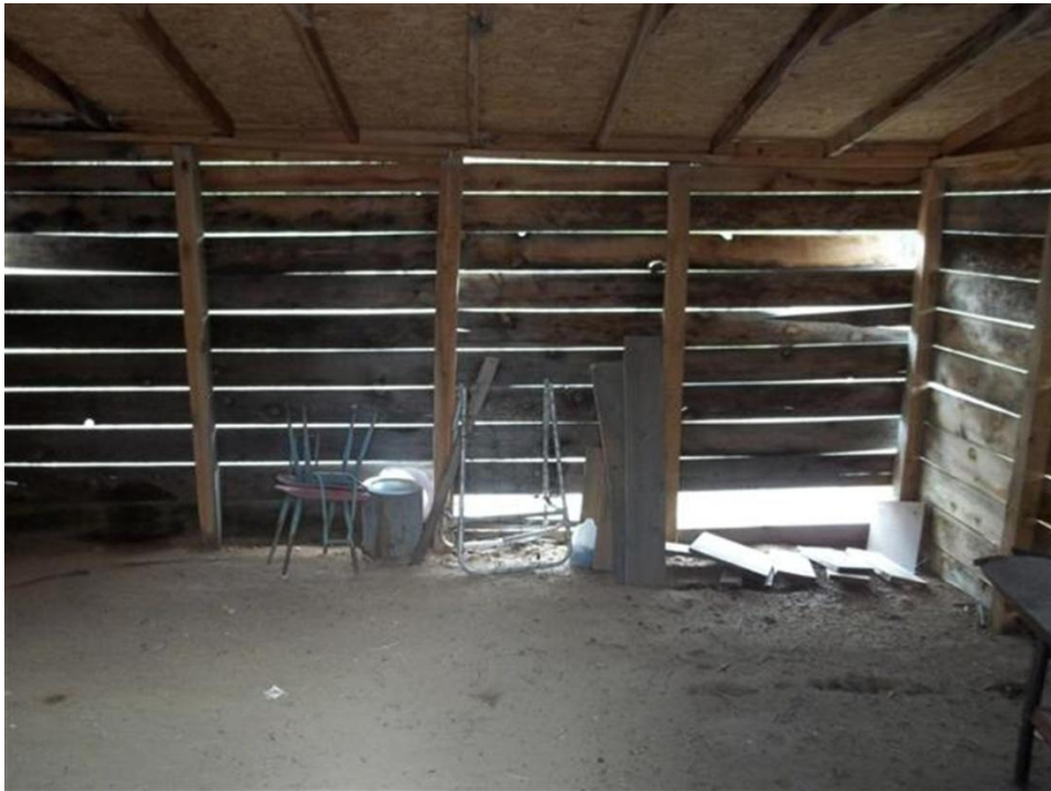
Photo 8: Mine Site #803; Nearby structure
