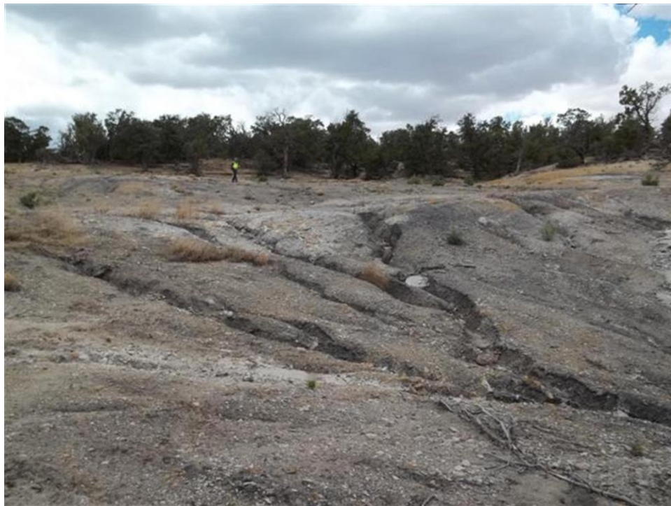
Photo 4: Mine Site #86; Erosion trenches
