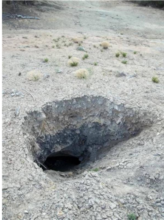
Photo 5: Mine Site #87; Possible collapsed adit/shaft
