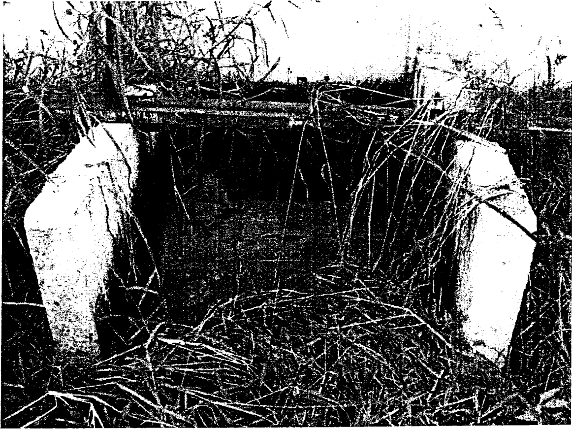
Barn 1 - full pit shown with liquid feed waste in manure, 9/19/05
