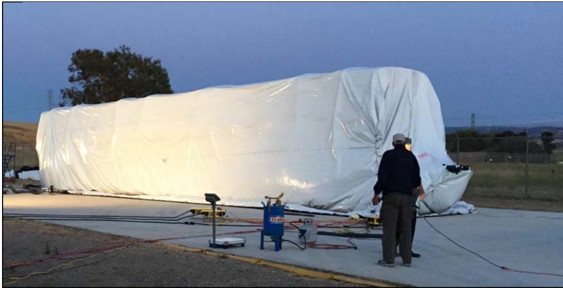
Figure 2. Tented railcar with HDPE tubing draped between the tarp and railcar visible as “ribs” under the tarp; MB scale and heater unit shown in foreground
