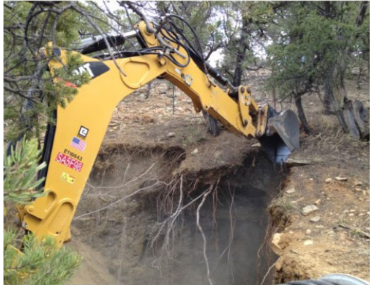
Closing of an Open Adit at Ruby #1
