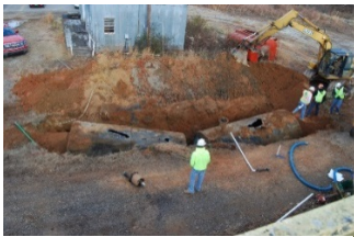
Removing USTs at former site
