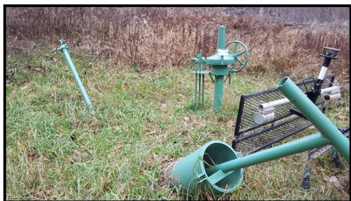
Leak rate quantified: Blow-down valve
