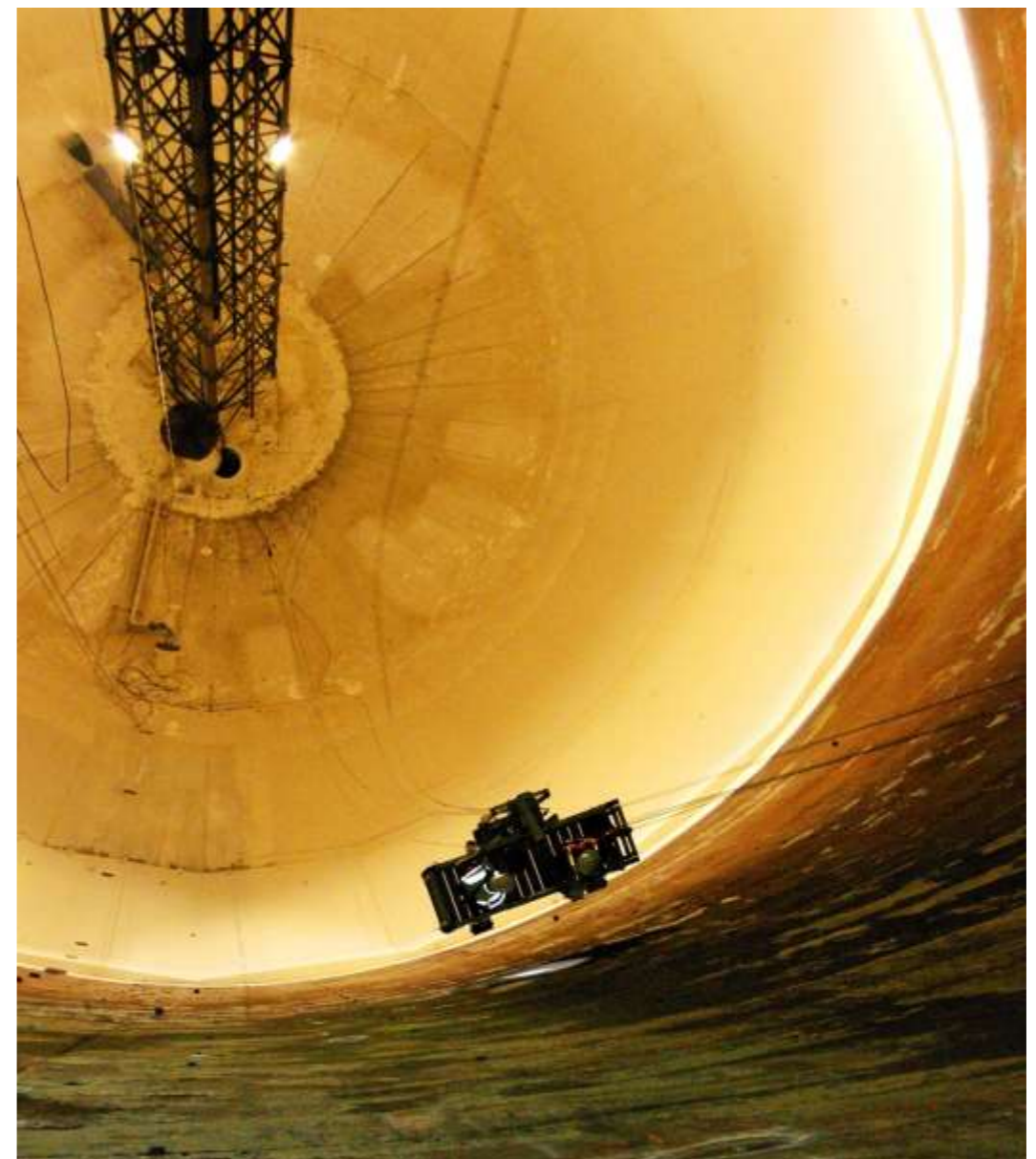
Work crew inspecting lower barrel of the fuel tank
