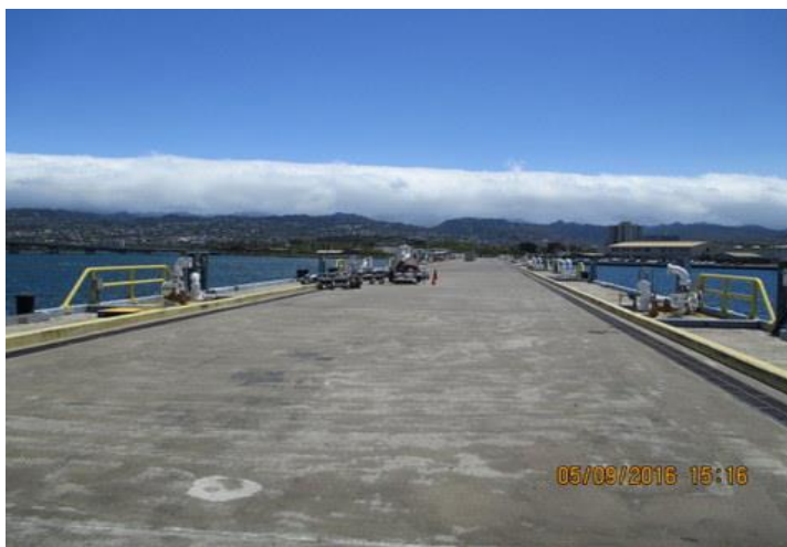
Figure 2. Overview Photo of the Hotel Pier
