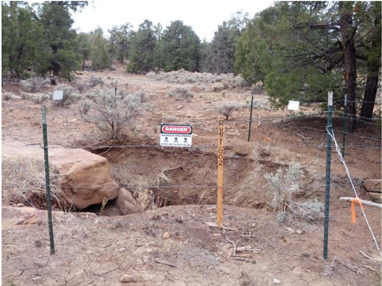
PHOTO 3: Ruby Mine #1 Vent opening and fencing, facing south.
