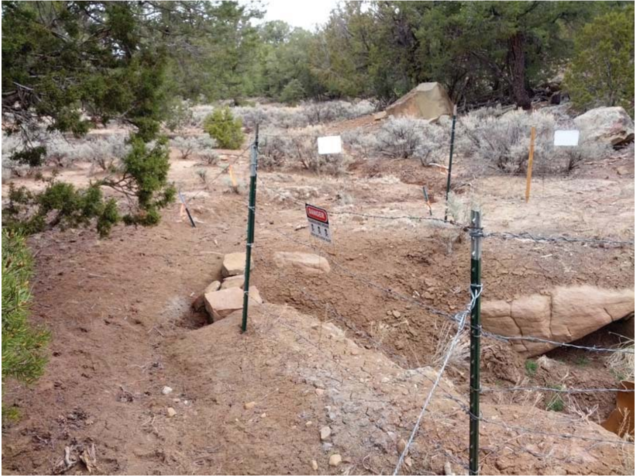
PHOTO 6: Ruby Mine #1 Vent fencing and warning signage, facing northeast.
