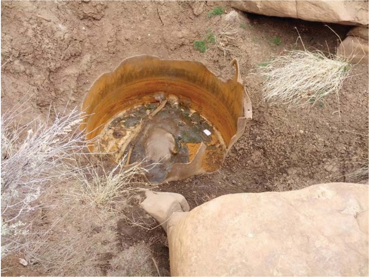
PHOTO 4: Ruby Mine #1 Vent taken from above. Note dead deer inside of vent.
