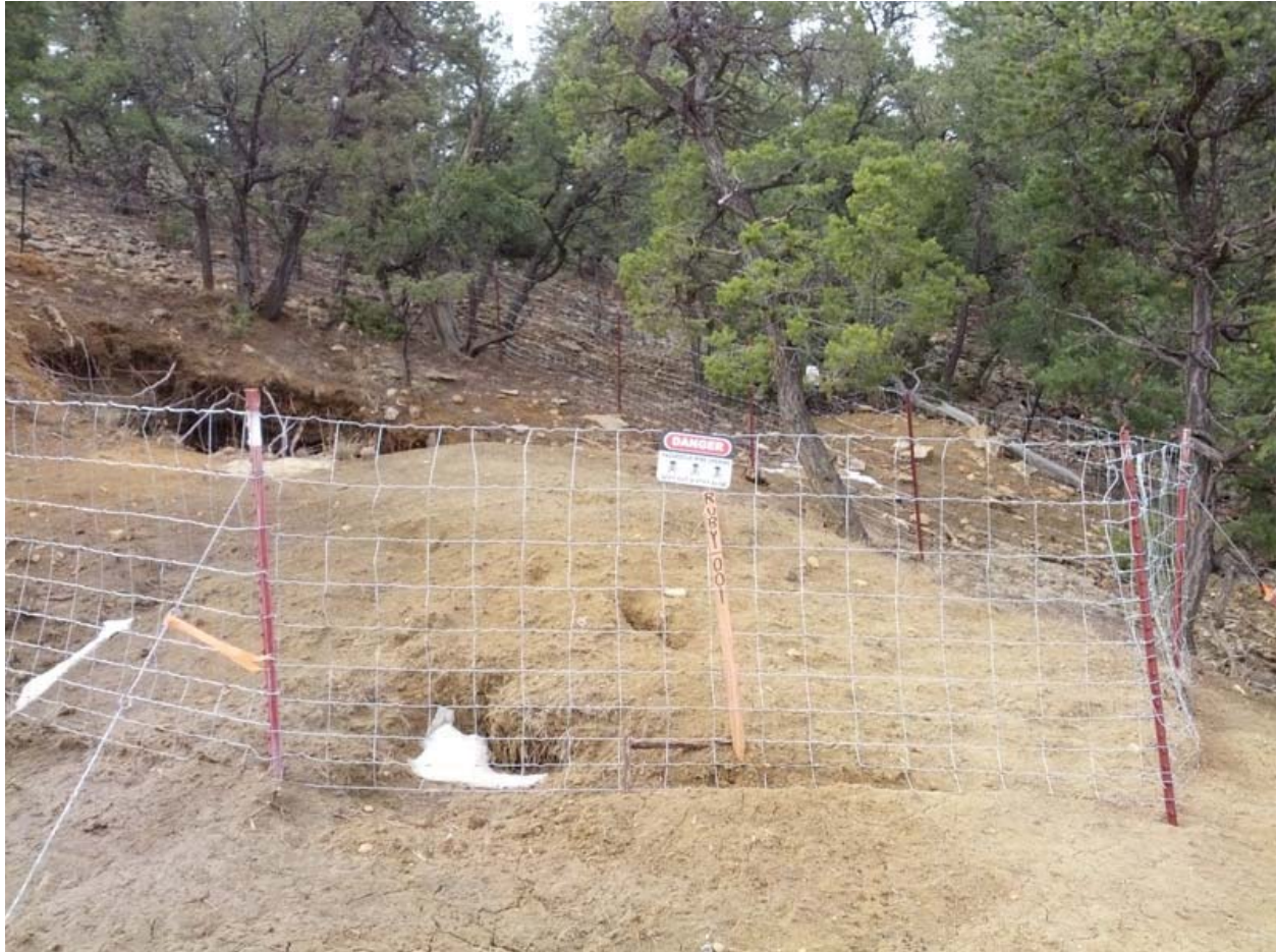
PHOTO 2: Ruby Mine #1 Adit fencing and warning signage, facing south. Small burrow visible next to stake.
