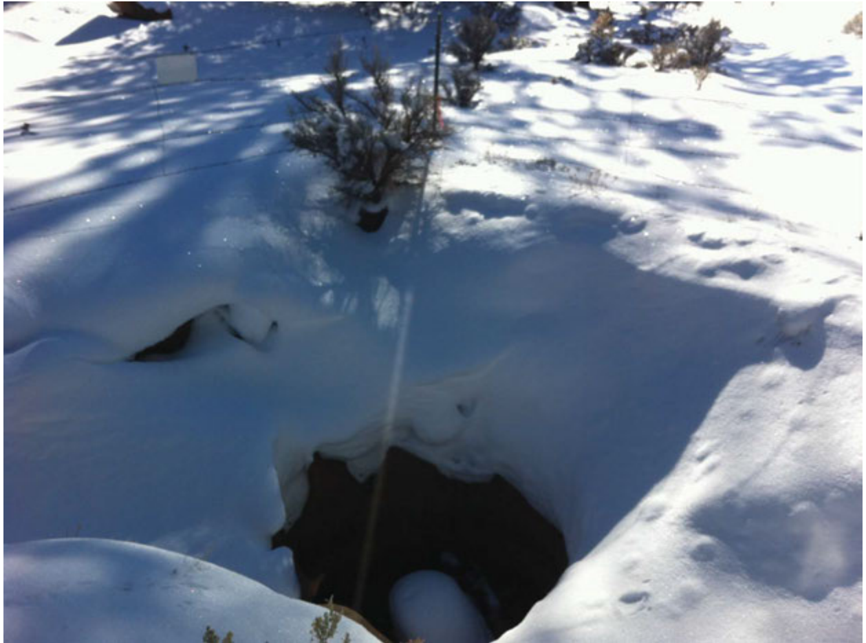
PHOTO 3: Ruby Mine #1 Vent opening and fencing, from north side of vent. Note water inside of vent frozen to 3'-4' bgs.
