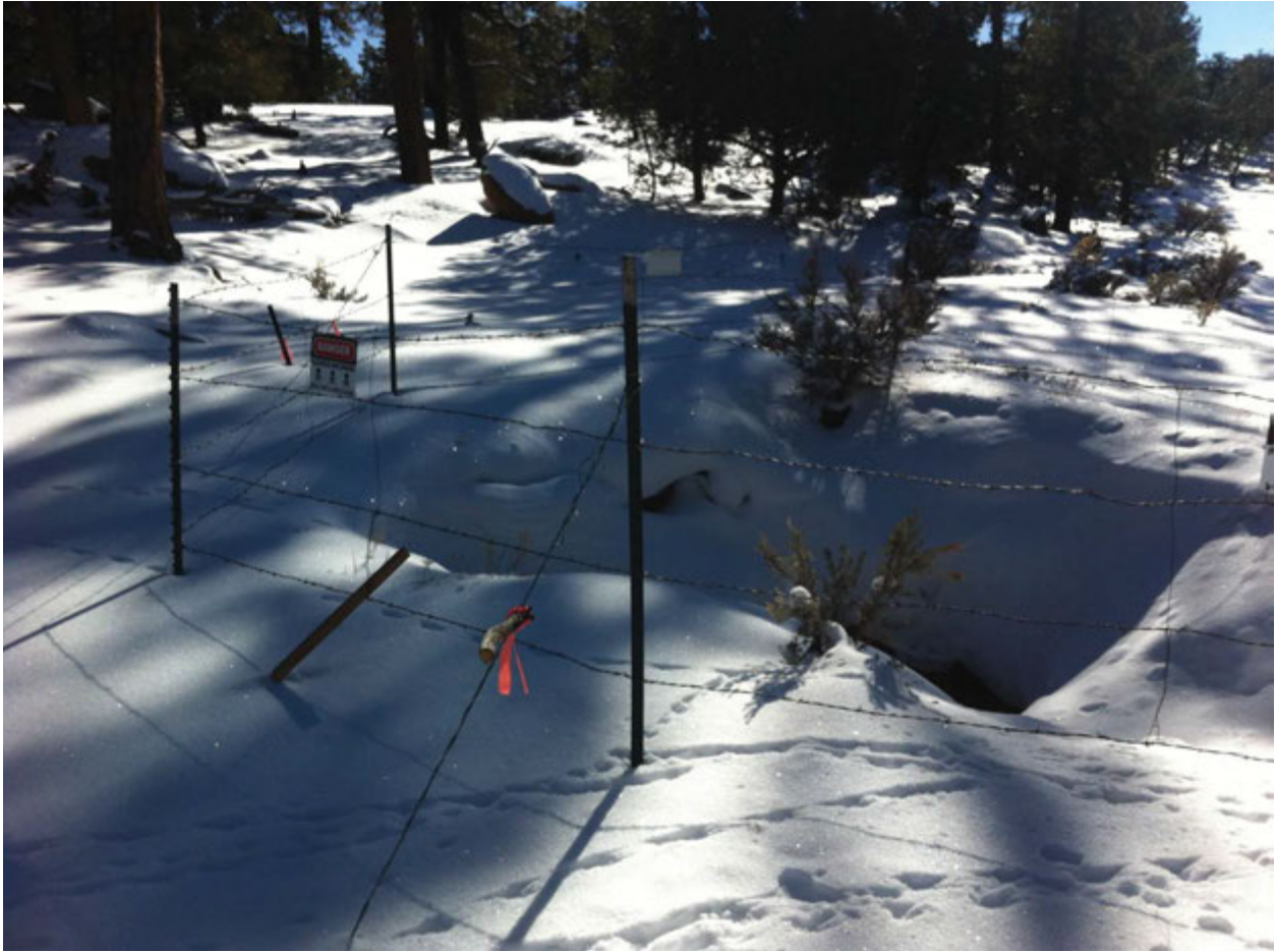
PHOTO 2: Ruby Mine #1 Vent fencing and warning signage, facing southeast.
