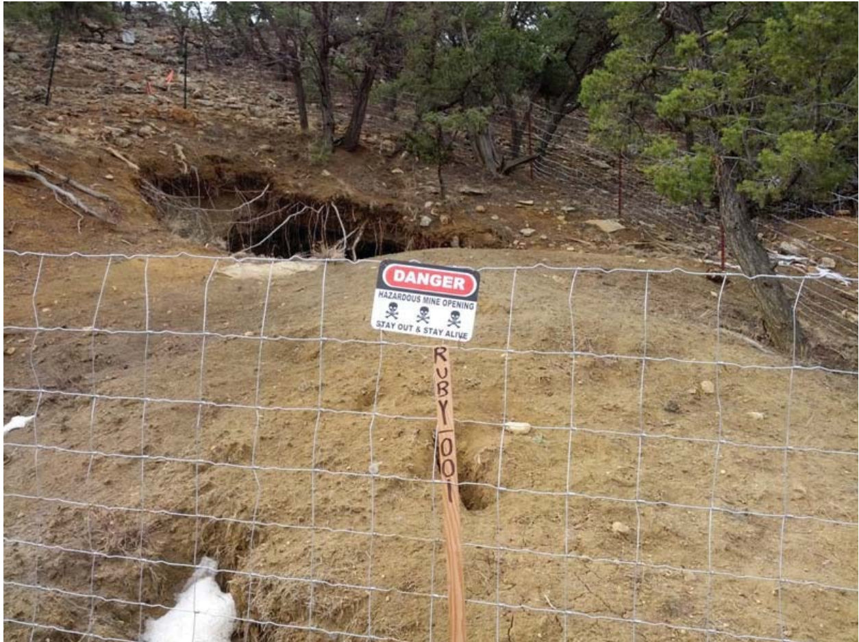
PHOTO 4: Ruby Mine #1 Adit warning sign and fencing. Facing south.
