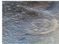
Monitoring well placed in the flow of surface run-off
