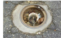
Monitoring well with missing cover and filled with debris
