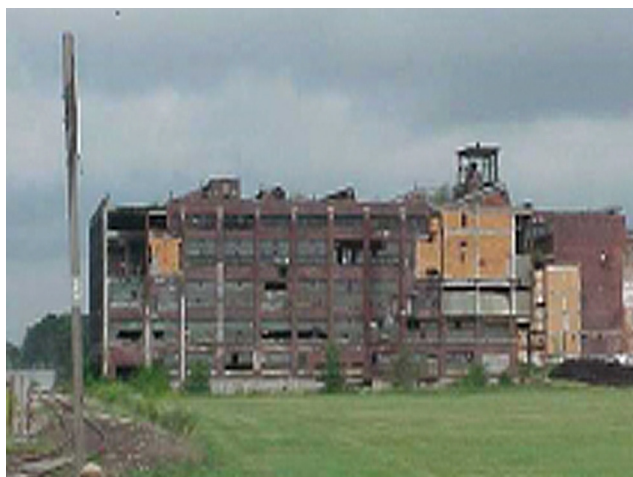
The Rath Packing Company plant prior to renovation, Waterloo, IA.
