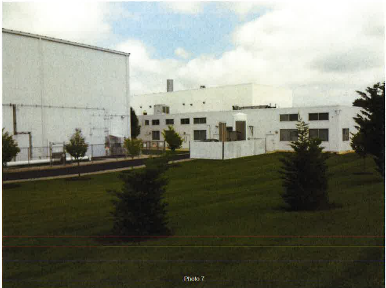
Photograph 7. SE corner of GMZ looking NW.
