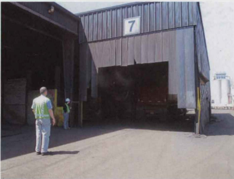
Photo 4. IMG_0349 at 11:22 am: Truck loading operations in Building 7. Note the fugitive dust escaping the enclosure.
