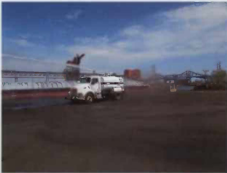
Photo 2. IMG_0347 at 11:05 am: SHB's watering truck onsite watering stockpiled material. SHB's water truck was onsite for the entirety of our inspection.
