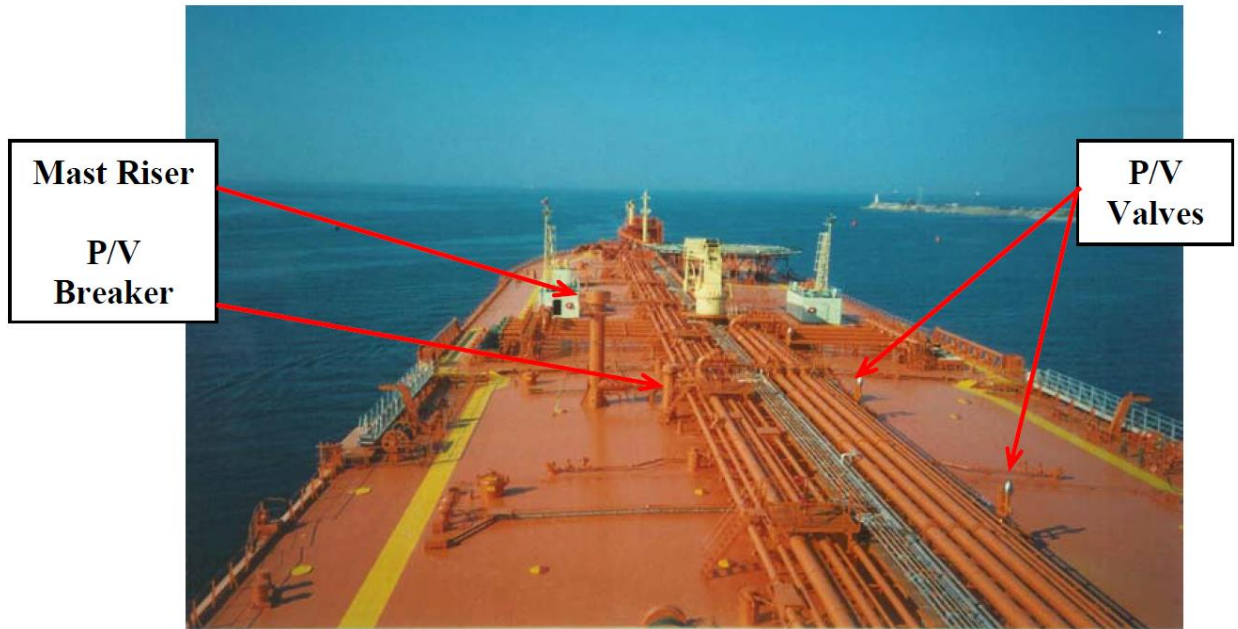
Figure 2-3. P/V valves, P/V breaker and mast riser on the deck of a tanker (source IMO MEPC.1 Circ 680 5 )
