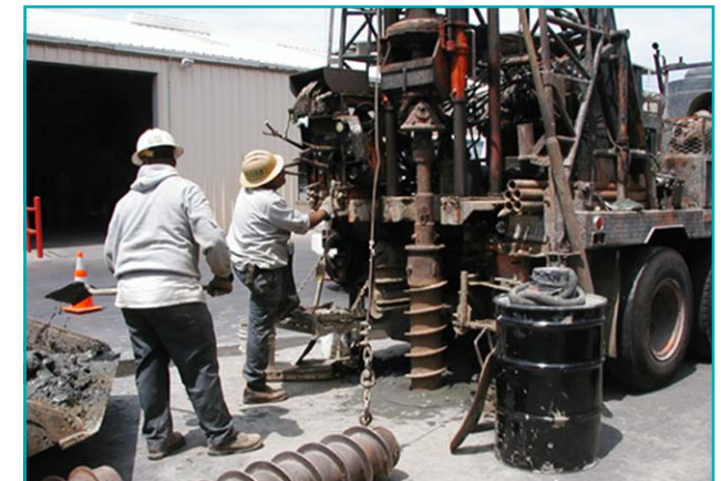
Installation of a monitoring well at Romic.
