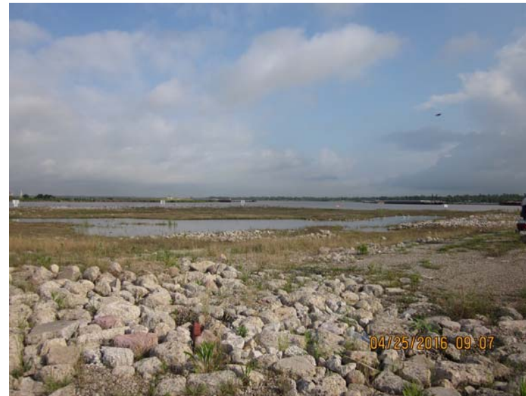
Photograph 20: Interior of Western Cell after heavy rainfall the week of April 18, 2016 (view northwest)
