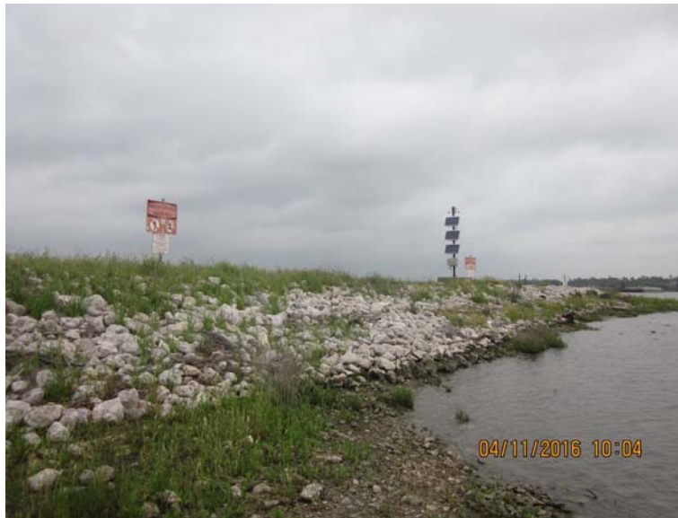
Photograph 07: Warning signs and security camera system along central berm (view northwest)
