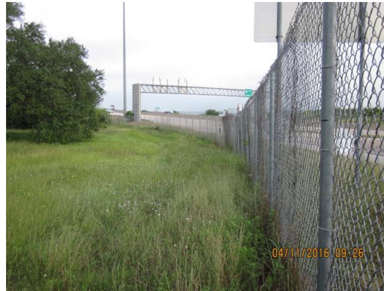
Photograph 16: Perimeter fencing on east bank south of I-10 (view northwest)
