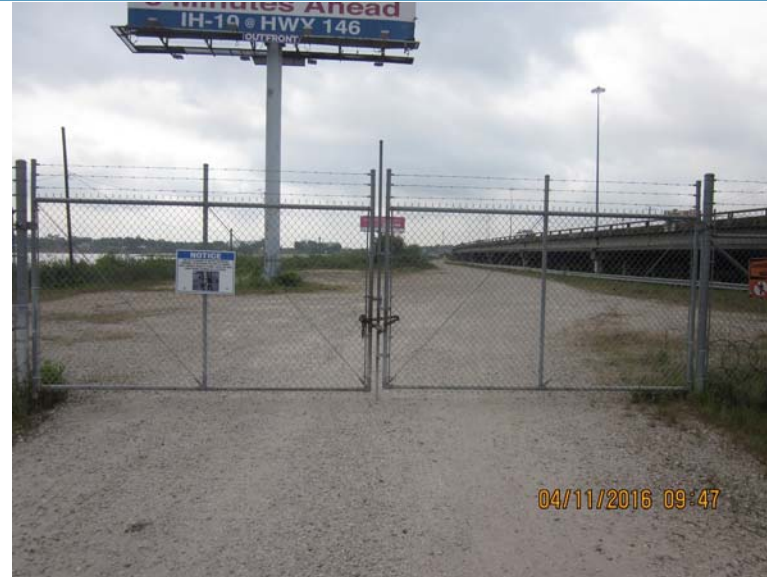
Photograph 02: Access gate north of I-10 (view east)
