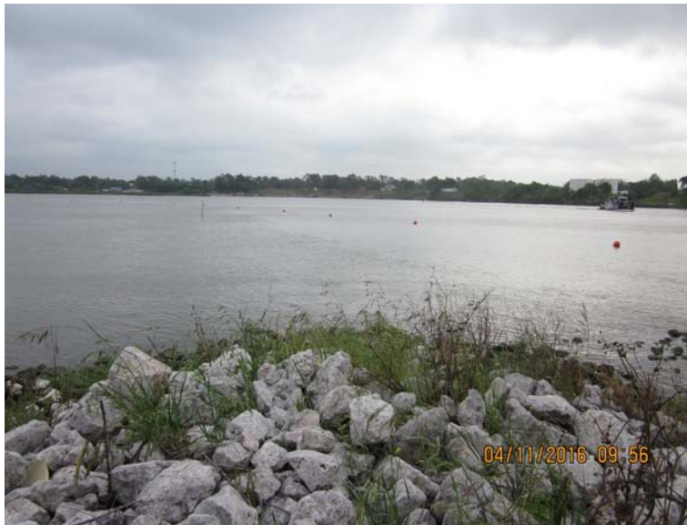
Photograph 03: Temporary buoys marking perimeter of Eastern Cell (view northeast)
