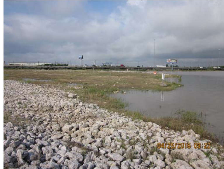
Photograph 22: Interior of Western Cell after heavy rainfall the week of April 18, 2016 (view southwest)
