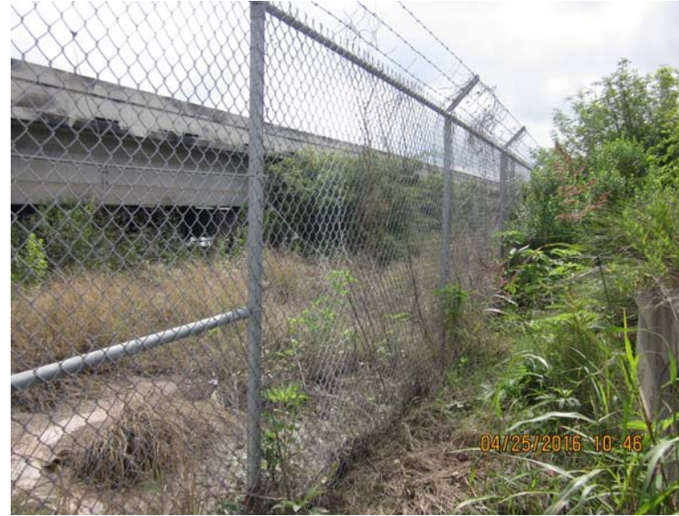
Photograph 14: Repaired perimeter fencing on west bank south of I-10 (view northeast)
