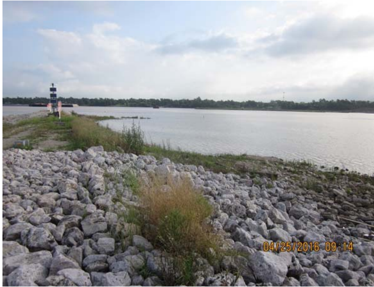
Photograph 21: Central berm after heavy rainfall the week of April 18, 2016 (view north)
