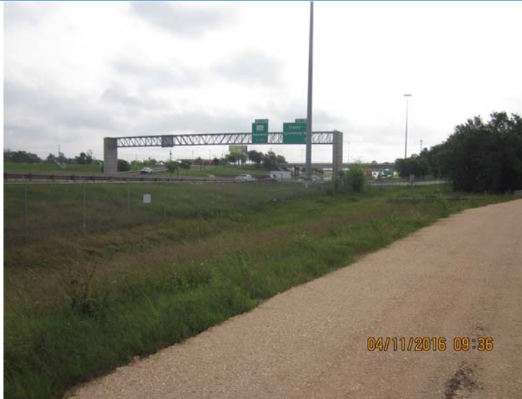
Photograph 17: Perimeter fencing on east bank south of I-10 (view northeast)
