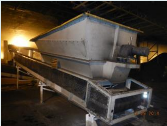
#23 / 24 Feeding Hopper Installation
