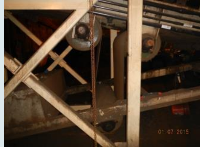
#24 Gravity Take-Up (GTU), Closer View
