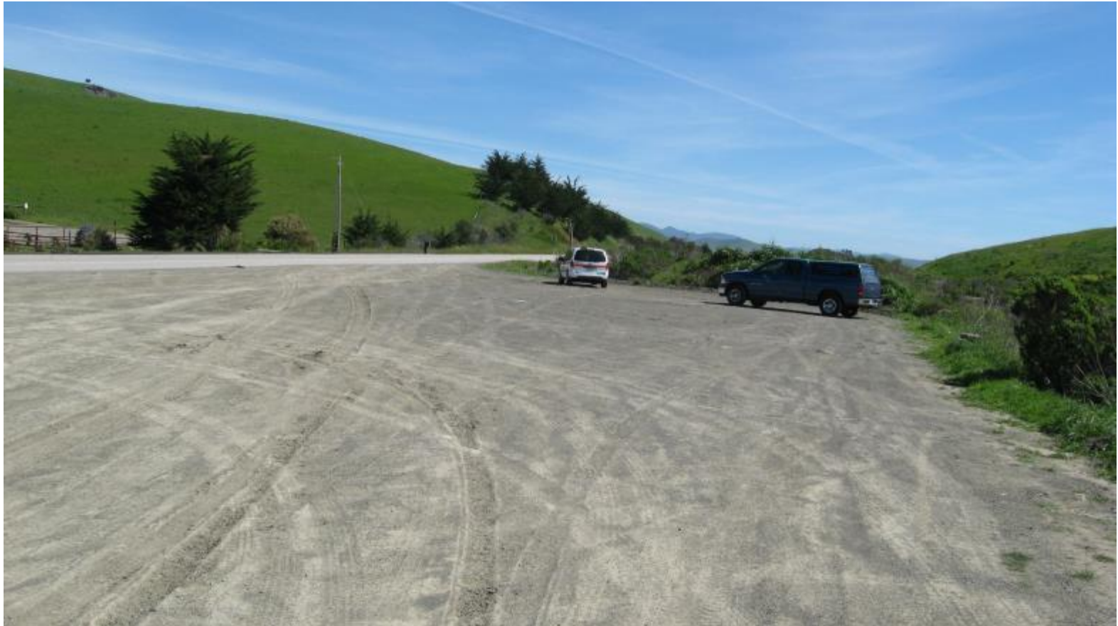
Before – Compacted roadside pullout
