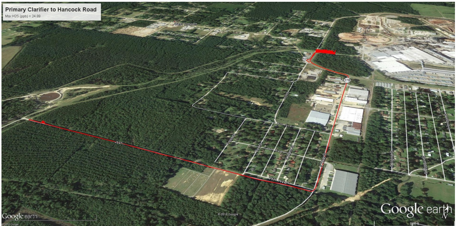
Figure 22: Concentration ribbon - transect - Primary Clarifier to Hancock Road (10/27/16)2
