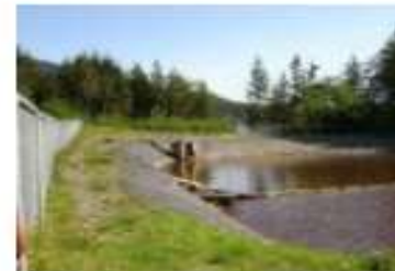
Figure 1. Landfill settling pond.
