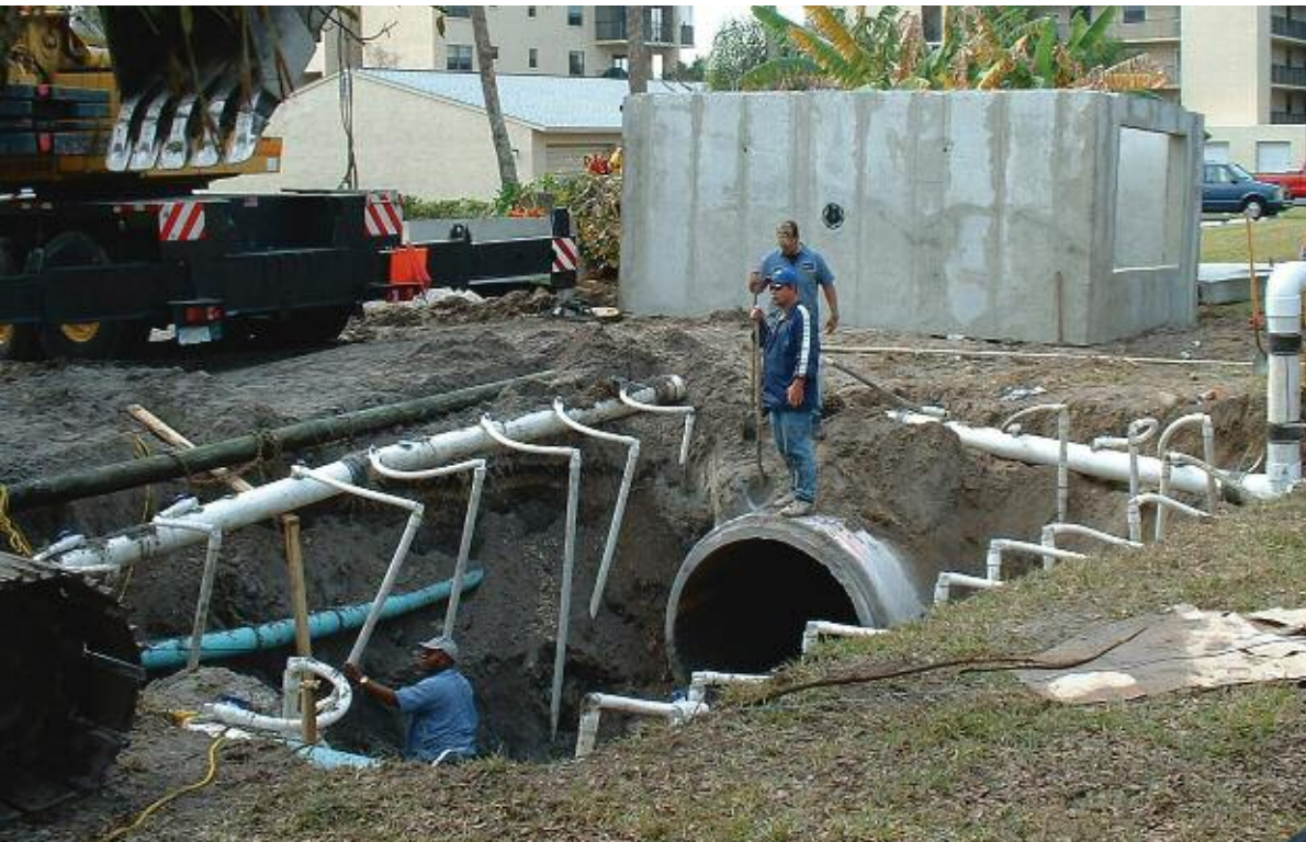
Large sediment traps like this one, near International Drive, have been installed throughout the city of Cape Canaveral to capture pollutants in the water before they reach the Indian River Lagoon.
