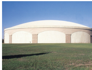
Above Ground Storage Tanks
