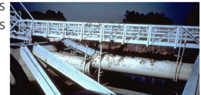
Damaged clarifier
