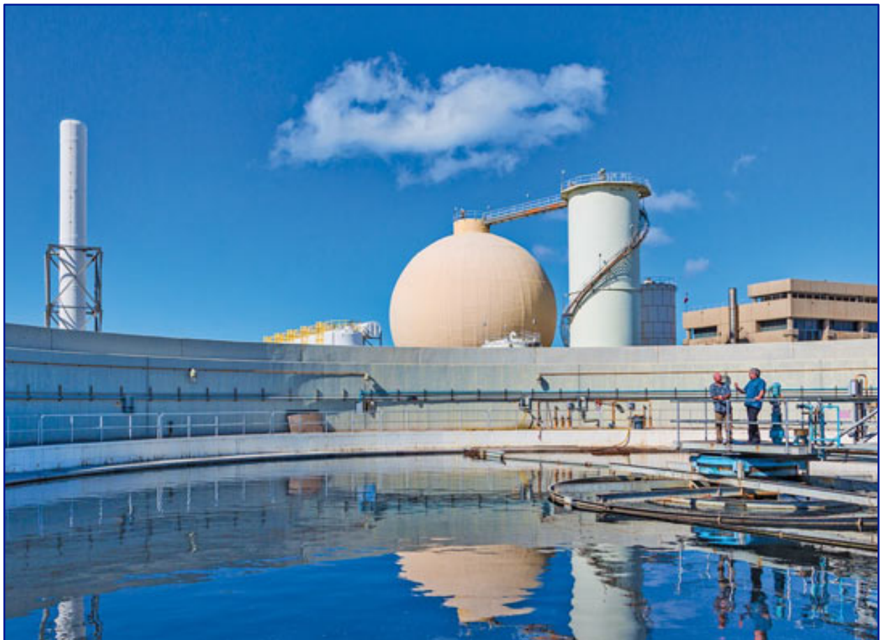
Honolulu's Sand Island Treatment Plant. Photo Source: American Infrastructure
