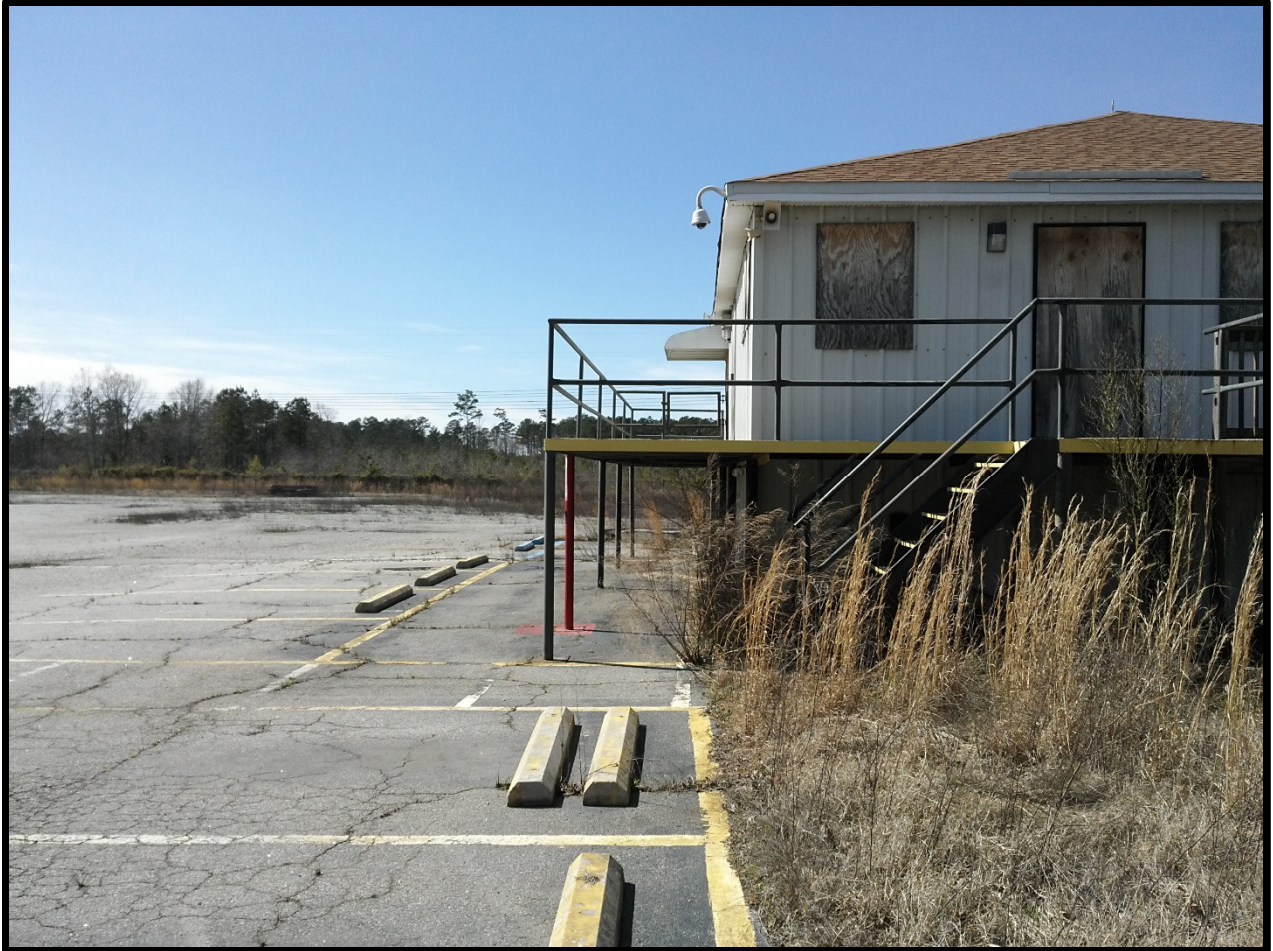
Picture 5: Office Building (East Direction)
