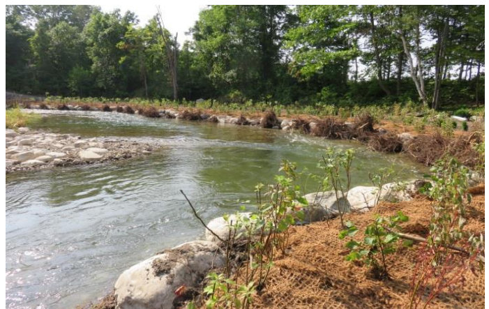
River restoration and tree planting at the Kagawong River (Manitoulin Island Stream Improvement Association).
