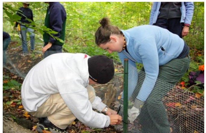
High school students erecting fence designed to keep reptiles off highway as part of a Lake Huron Youth Summit (ECCC).
