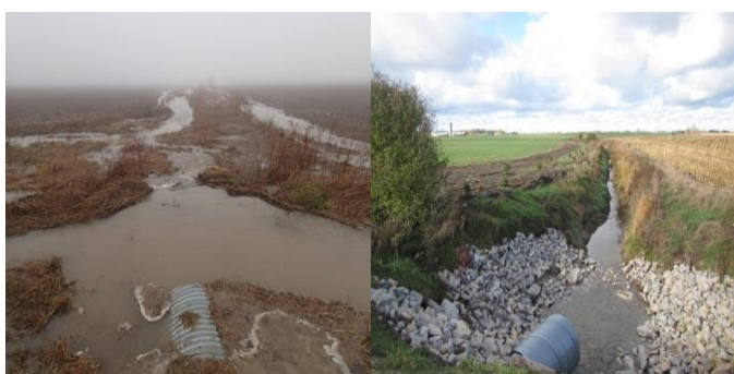
Before and after ditch and sediment trap as part of municipal drain project (Maitland Valley Conservation Authority).
