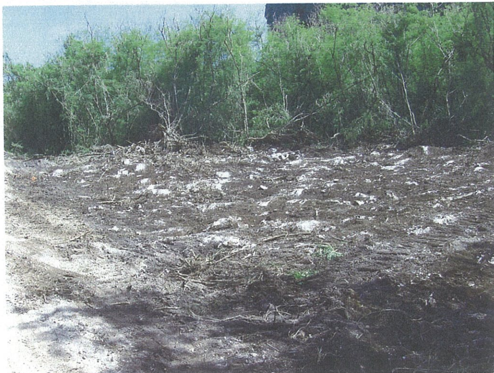
Drill Site Preparation – Note Extensive Rock
