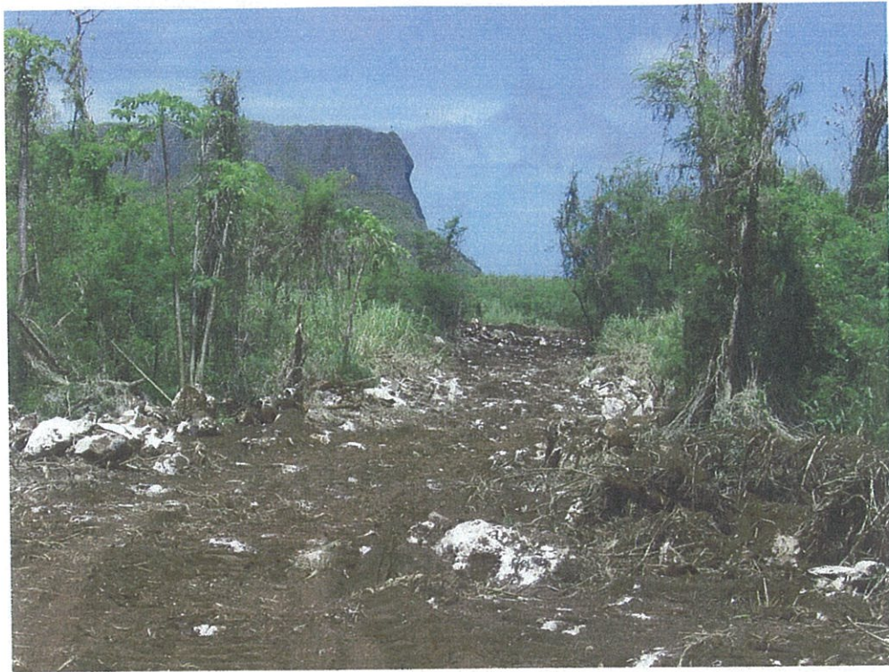
Access Road Initial Mucking & Clearing
