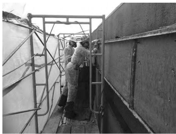
Interior poly and tape being installed to seal the work area for negative enclosure.
