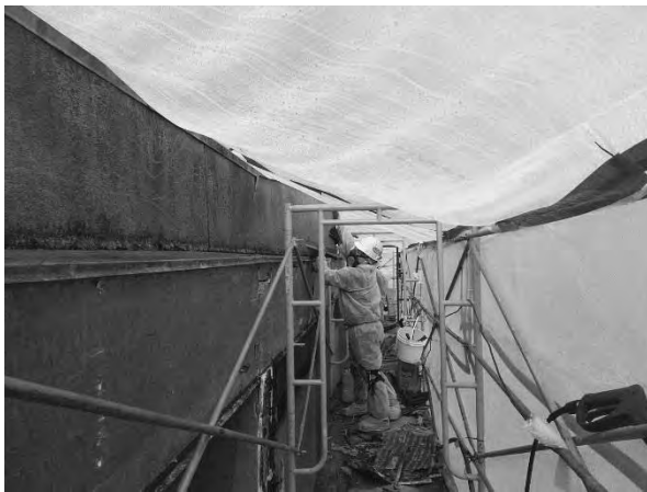
Interior poly and tape being installed to seal the work area for negative enclosure.
