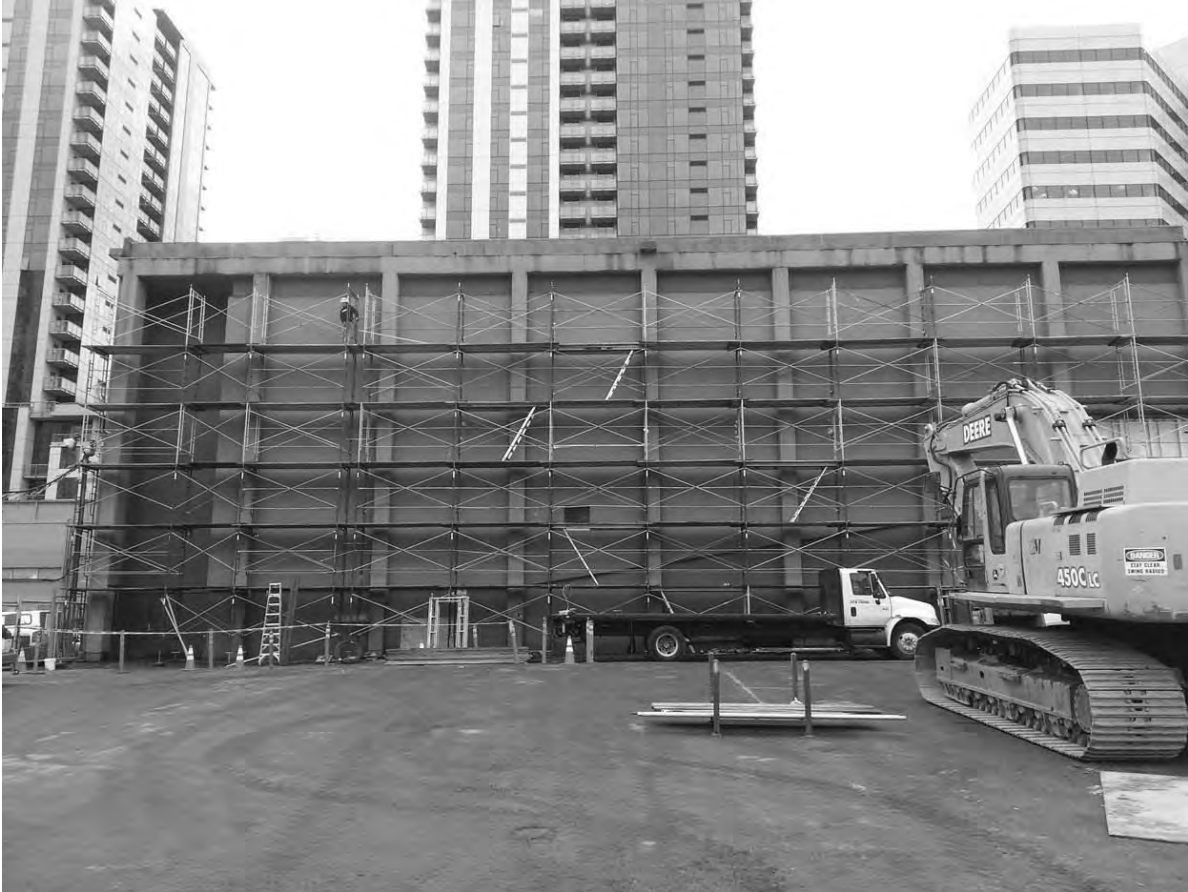
Example of scaffolding being erected
