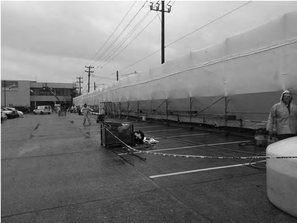
Final wrap of scaffolding
