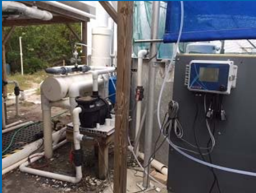
Mote Patented Ozonation system used for Marine Mammal Hospital
