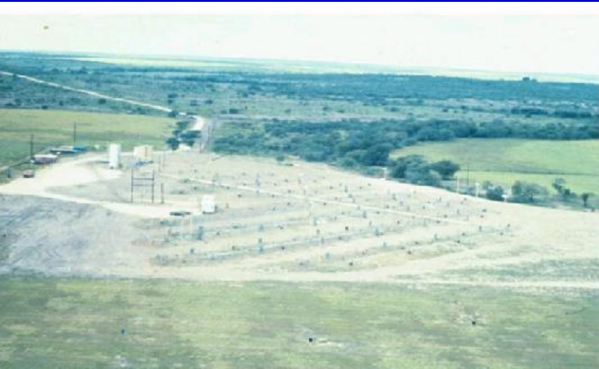
In situ wellfield with numerous injection and extraction wells
