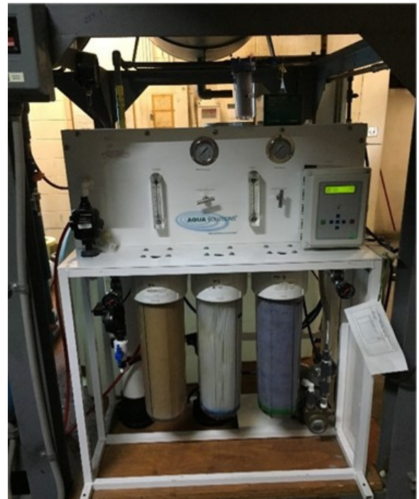
Figure 7. Centralized RO systems produce deionized water for research purposes in the main building and TERF.
