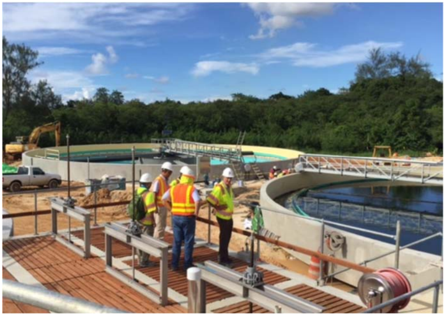
Photo 6: New WWTP at Agat-Santa Rita in Guam
