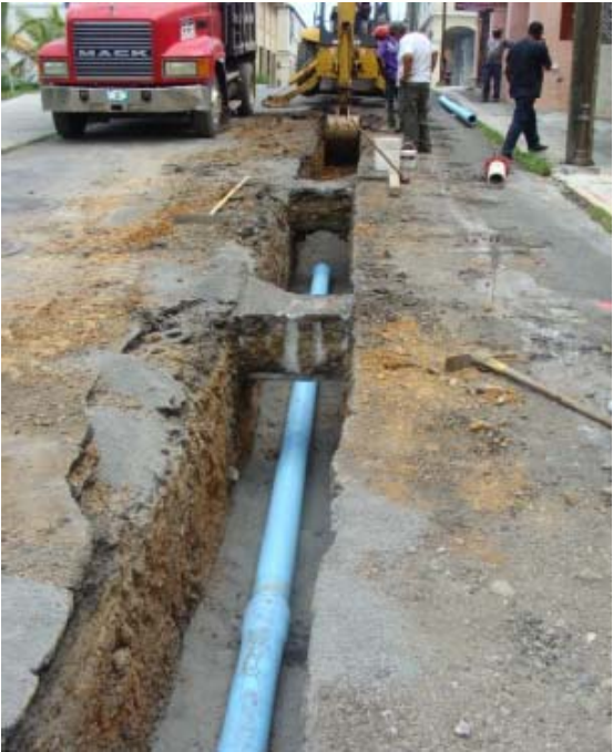
Photo 1: Christiansted Waterline Rehabilitation Project (photo courtesy of Harold Mark, VIDPNR)
