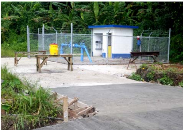
Photo 4: Drinking Water Infrastructure Improvements (photo courtesy of ASPA)
