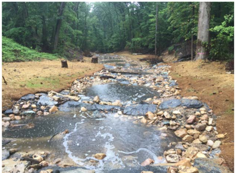
Photo 2: Alger Park Stream Restoration (photo courtesy of Josh Burch, DOEE)
