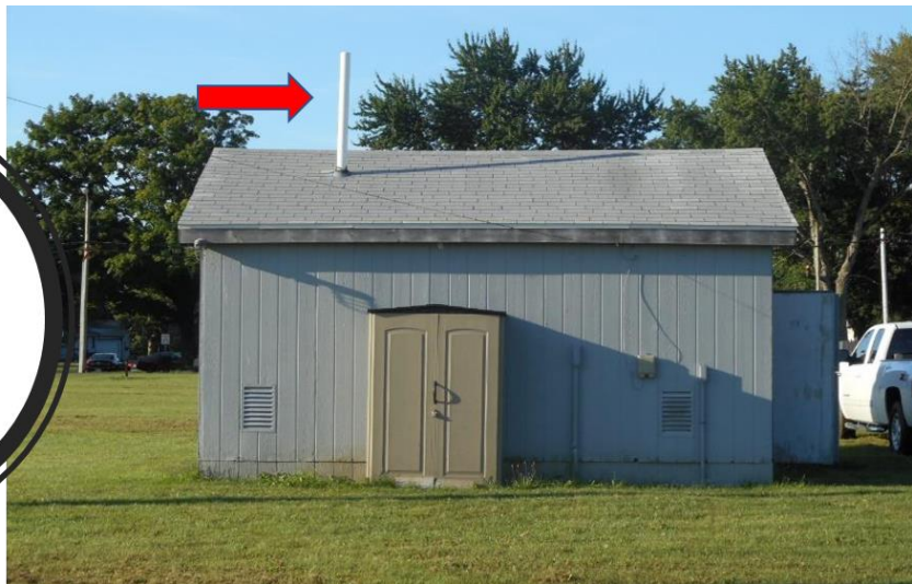
Figure 1 – Groundwater treatment building on the former Amphenol site.
