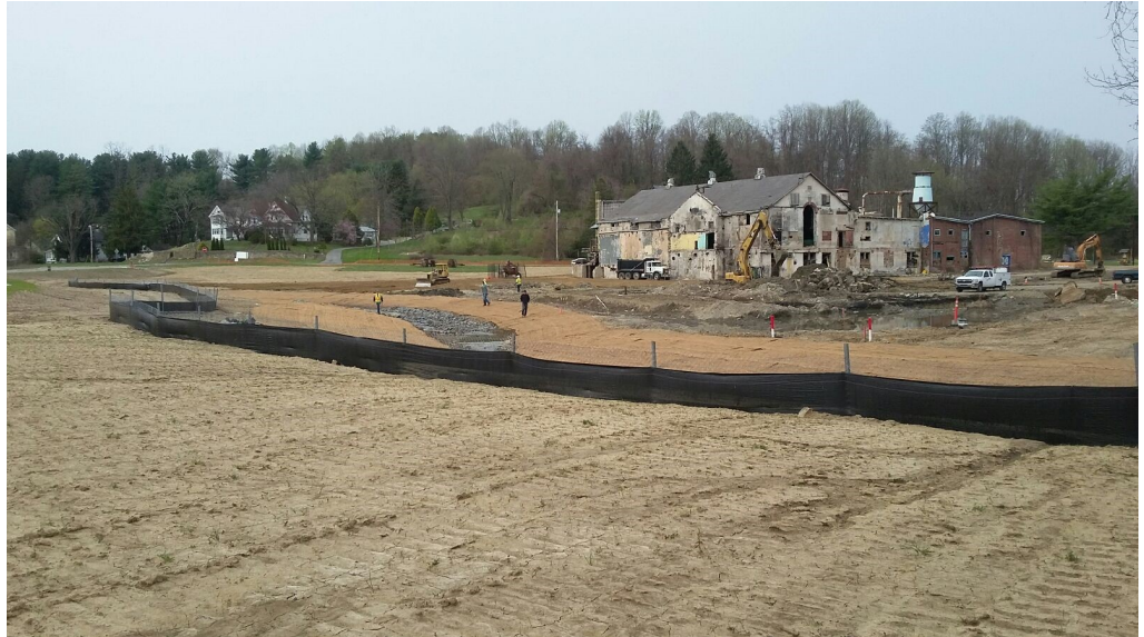
Construction at the former Marshall Brothers Paper Mill.
