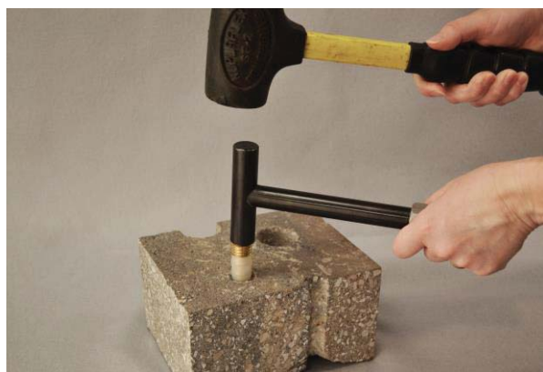
Figure 2. Installing the Vapor Pin™.
