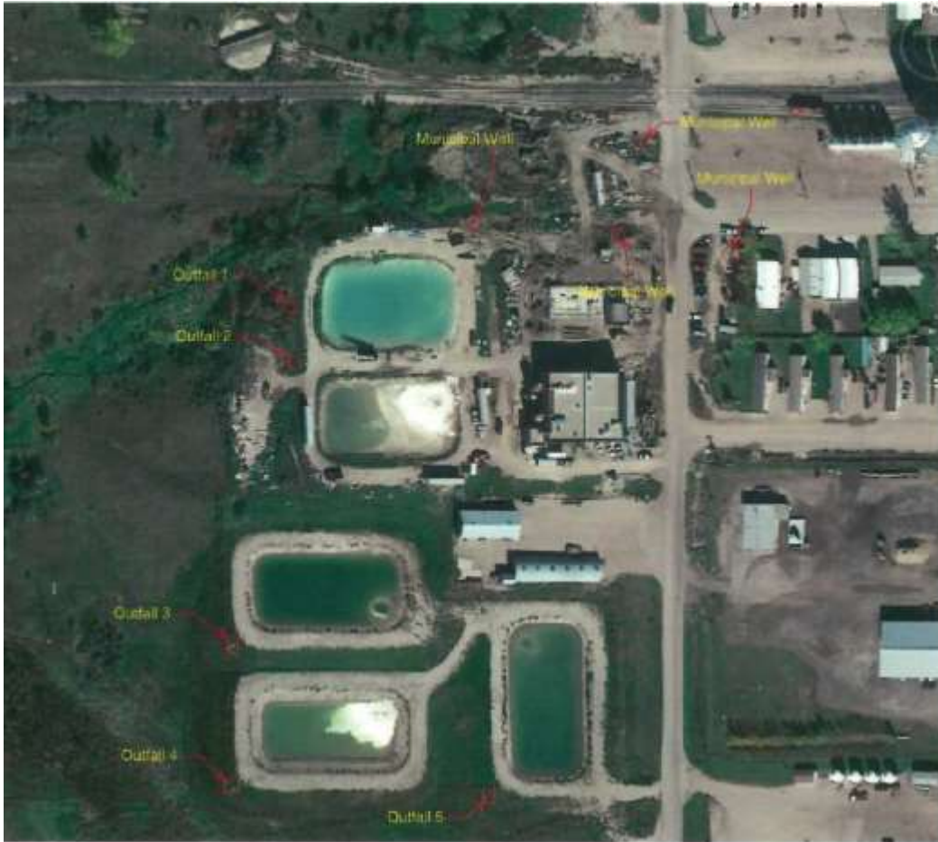
Figure 1 - Overhead Photograph of New Town Water treatment plant and Lagoon system with outfall points identified
