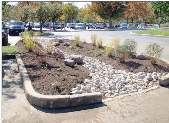
Figure 2. Completed rain garden at Subaru of America in Cherry Hill, New Jersey.
