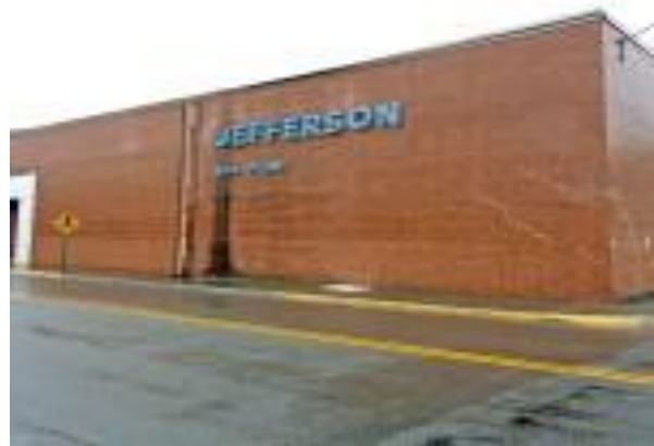
The Jefferson Yards Hill Plant on Valley Street was once a booming textile industry but has not been used in recent years.
