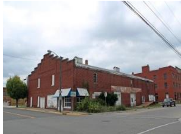
The former Virginia Wood Products Building, which was torn down in 2015 for redevelopment
