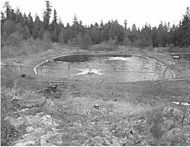
1.Primary Lagoon with 2 aerators
