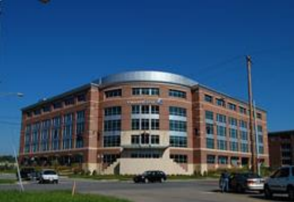
Virginia Tech's Carilion School of Medicine. The school's first class entered in the fall of 2010, only days after the building was constructed.
