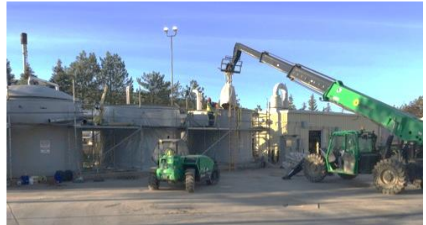
Iron sponge media being loaded into vessels
