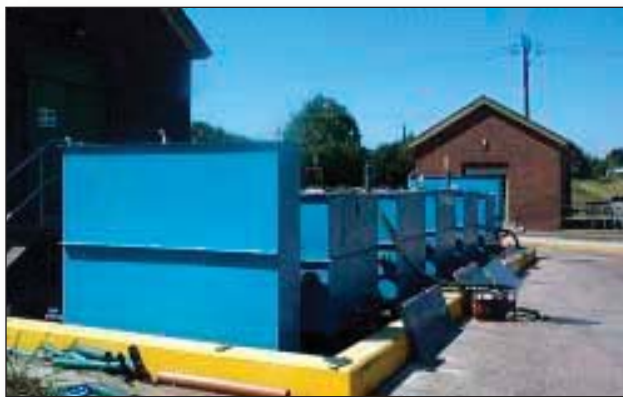
ABR installation. Photo courtesy of Atkins Water, 2006.
